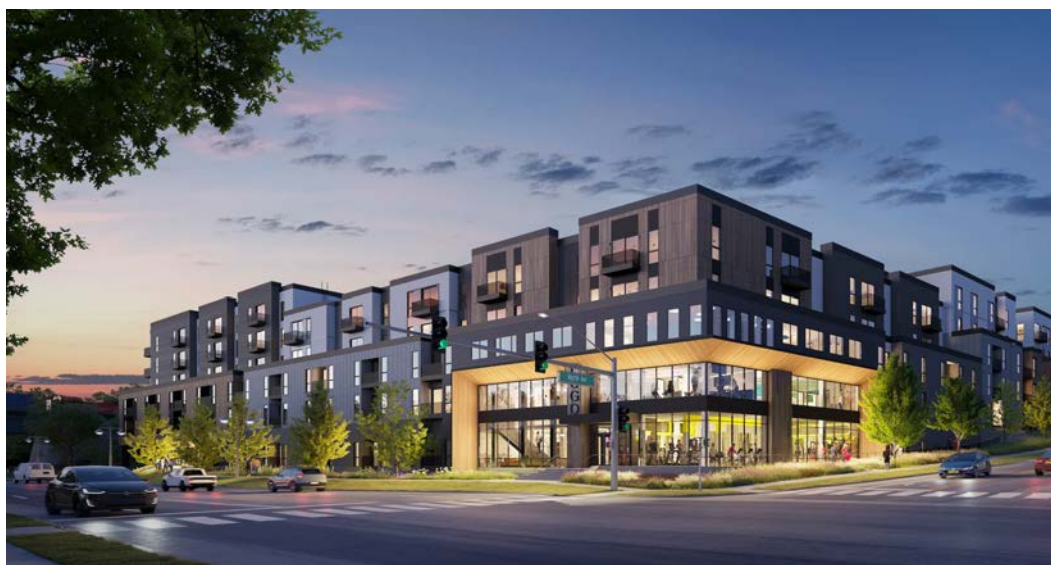
Replay student housing located at the intersection of S. Riverside Drive and Myrtle Street opens in Fall 2025 with 291 fully furnished units.
