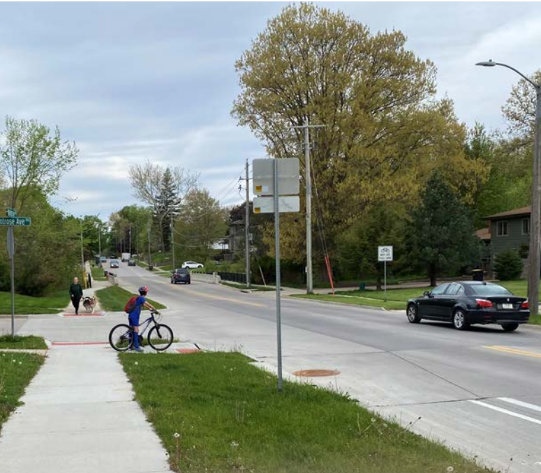
As part Iowa City’s Complete Streets Policy, bicycle lanes are considered whenever arterial streets are reconstructed or extended. The image above shows new bike lanes on Rochester Avenue.
