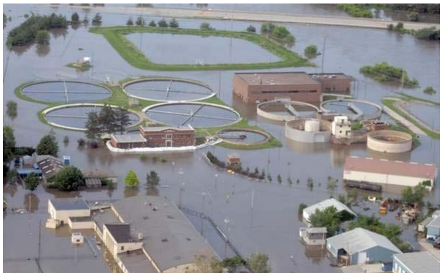
A view of the City's North Wastewater Treatment Plant, surrounded by floodwaters last June.
